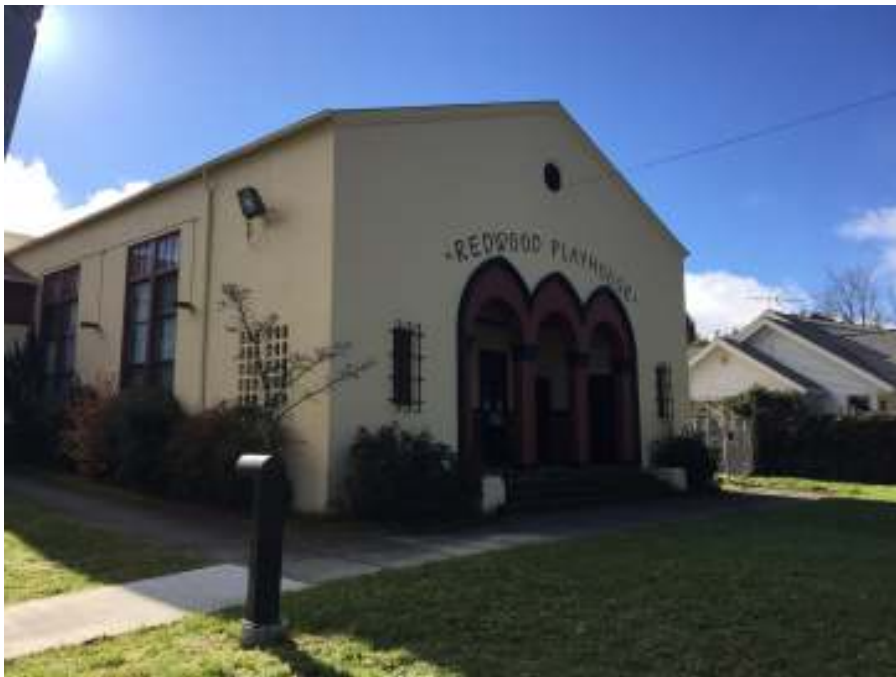
View of school building looking southwest.
