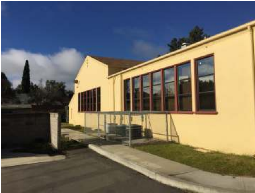
View of school building looking west.
